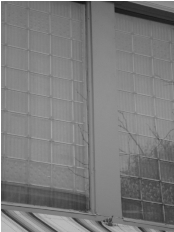
Figure 8 This storefront (322 East Lake Street) still retains its original transom. To improve energy efficiency an outer storm window has been added.
