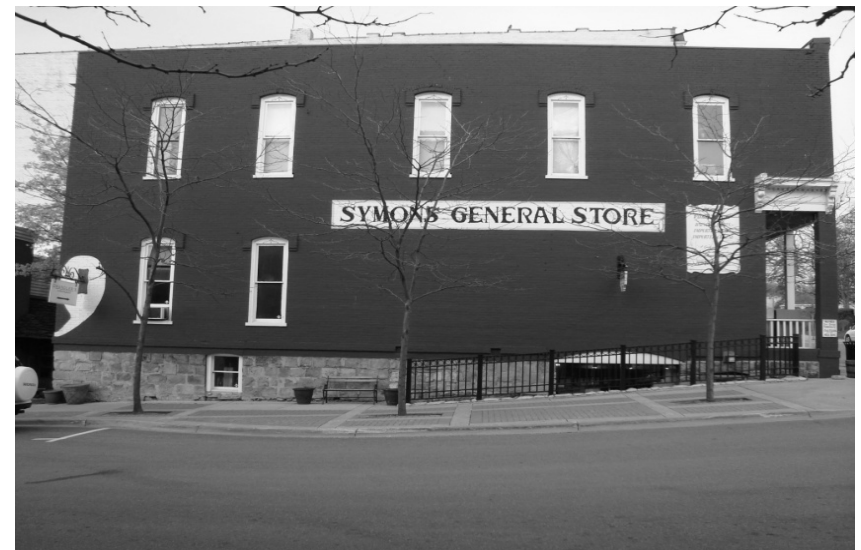
Figure 27 Historically one elevation of corner buildings had to be the load bearing wall (401 East Lake Street)
