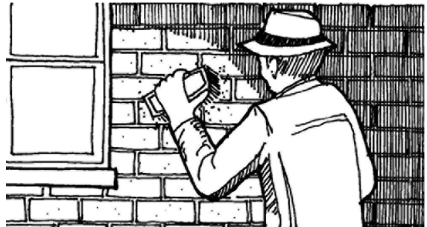
Figure 2 Use a soft bristle brush when scrubbing masonry
