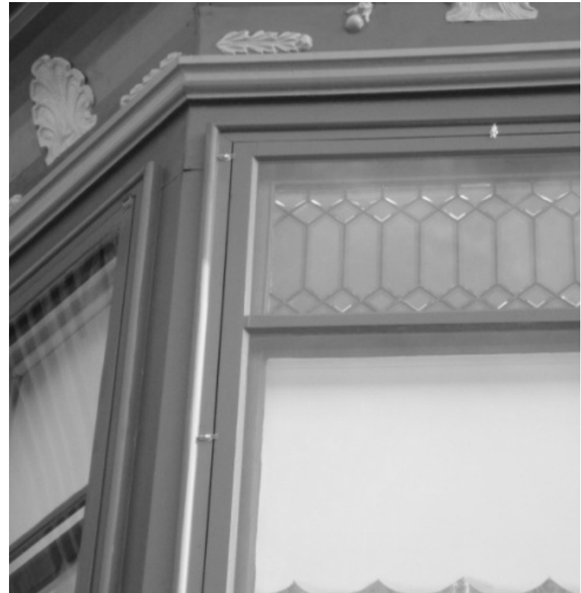
Figure 7 This building used an exterior mounted storm window to achieve a higher thermal efficiency. Calumet, MI
